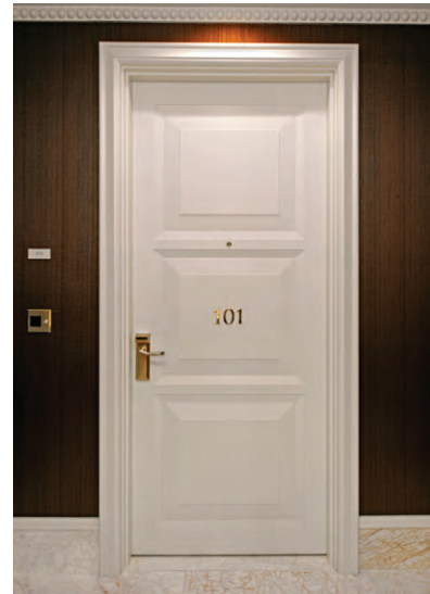
20-minute fire-rated TS3000 in MDF
