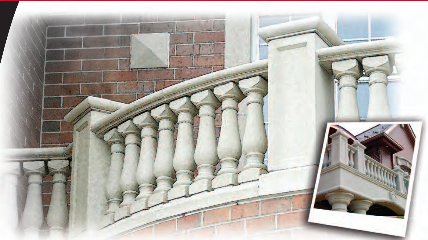
Plain view of top rail and piers.
