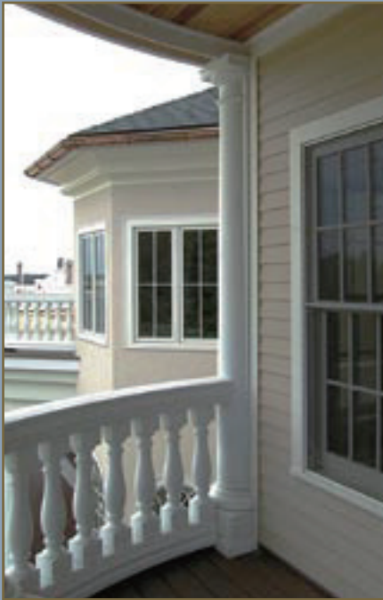
Photo above illustrates the use of the following Spectris products: baluster BAL 2000-25 and curved rail RAL 2100 top & bottom.
