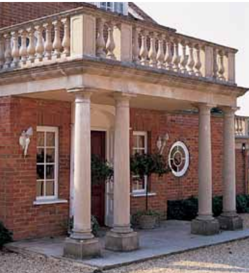
Portico D, M7 Columns and Balustrading.
