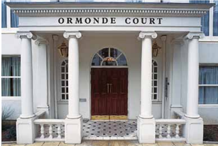
M4 Columns on special Piers with L210 Upper Cornice, L220 Lower Cornice and L330 Architrave
