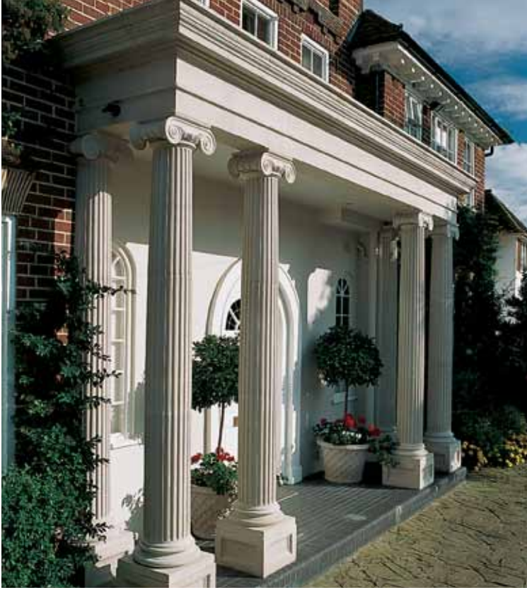
Portico A with M2 Columns.
