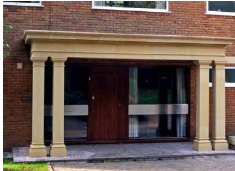
Portico A with square M7 Columns.
