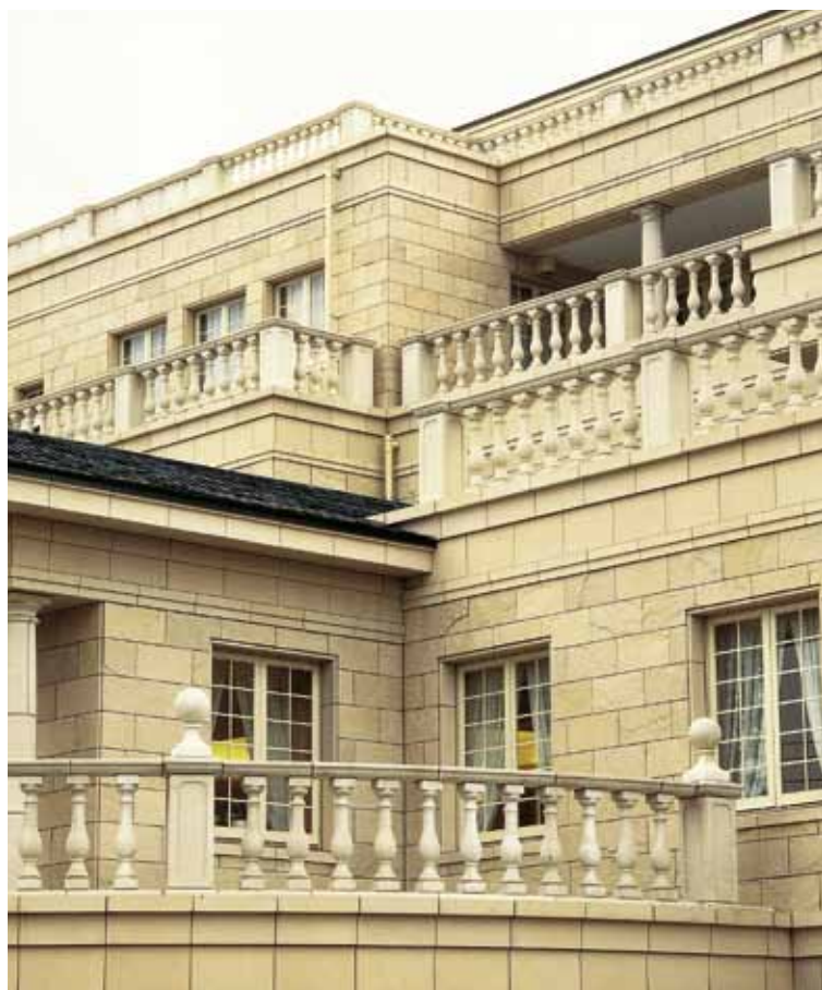
Hospital in Japan makes extensive use of custom and standard Haddonstone.
