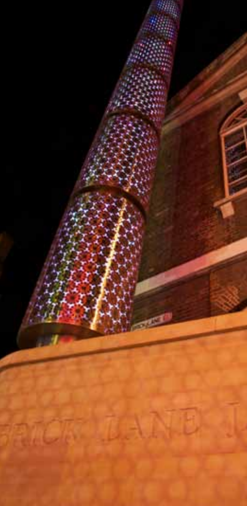
Custom cladding at Brick Lane Mosque, London.
