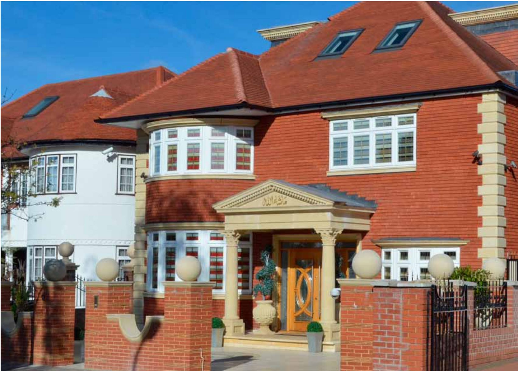
London residence transformed by incorporating Haddonstone architectural features including custom portico, window heads and cills, quoins, copings and balls.
