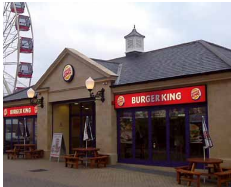
Extensive use of custom cladding for prominent fast-food outlet in Bridlington.
