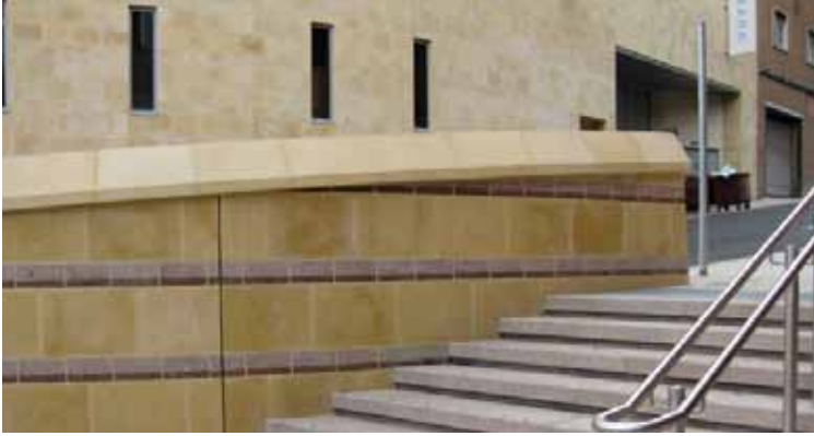
Londonderry city centre features extensive cladding by Haddonstone.
