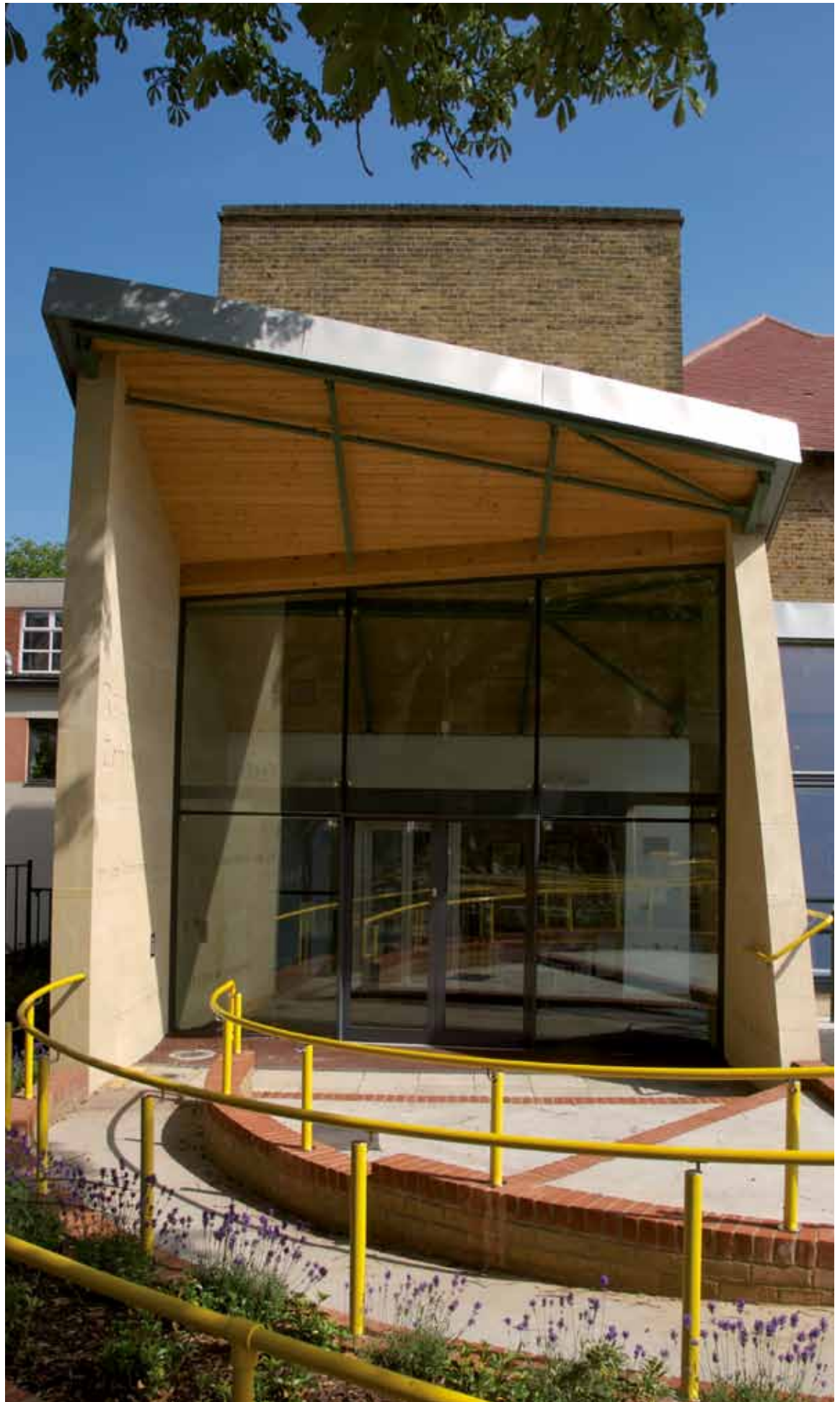
The dramatic entranceway to The Rutherford Centre for the Performing Arts at Wimbledon High School utilises custom cladding from Haddonstone.
