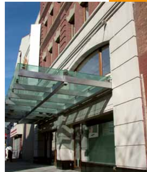
Cladding on a New York Development.
