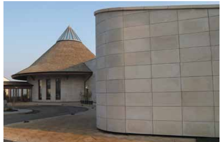
Rain screen cladding at Seaham Hall Hotel and Serenity Spa.
