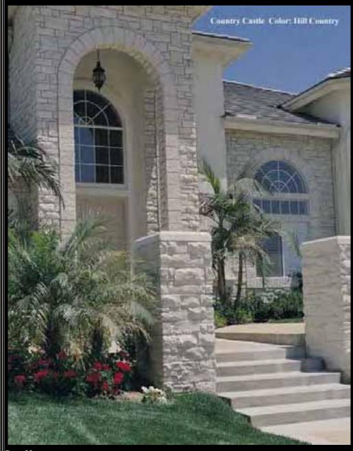
The design for Country Castle was inspired by the natural saw-cut chiseled limestone in a true ashlar pattern. Sizes range from 1 1/2" to 8" in height and from 4" to 20" in length.
