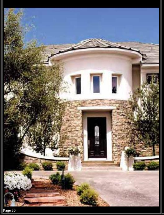
Country Rubble is an ashlar pattern stone with hand hewn style edges for a rustic effect. Country Rubble can be installed with tight fitted joints or with a mortar joint. Sizes range from 2" to 10" in height and up to 23" in length.
