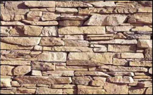
Square foot coverage for Eastern Ledge is based on installation with ½" mortar joints.
