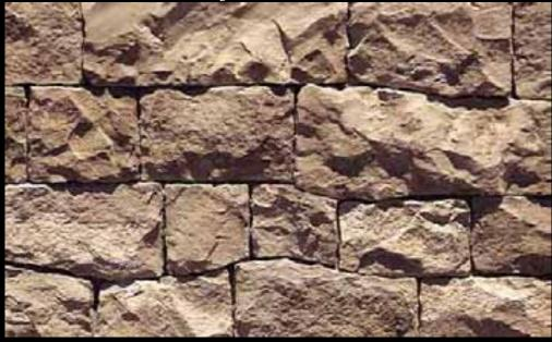
Square foot coverage for Carolina Rubble is based on installation with a ½" mortar joint. Page 37
