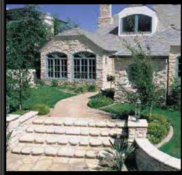
Coronado was the first to manufacture Mountain Ledge over 23 years ago. Mountain Ledge is comprised of individual stones with an average thickness of one to three inches. Stones range in size from 1" to 4" in height and up to 20" in length.
