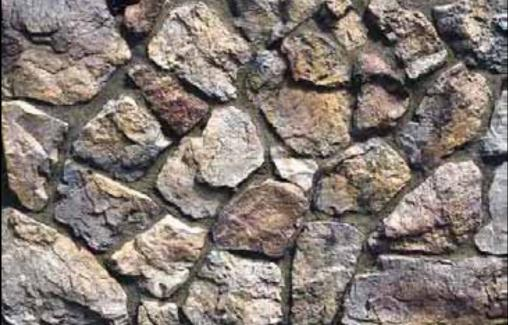
Square foot coverage for Villa Stone is based on installation with a 1/2" mortar joint. Page 9
