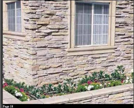
**Virginia Ledge** is a combination of 2" and 4" stones. The two sizes make Coronado's panels very difficult to detect. The thickness of Virginia Ledge varies from 1" to 3" creating a more "rugged" look as compared to Quick Stack.
