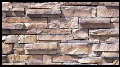
Square foot coverage for Idaho Drystack is based on installation with tight fitted joints. Page 27
