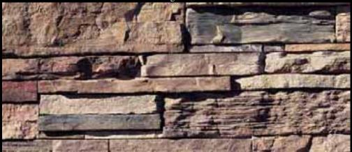
Square foot coverage for Weathered Edge is based on installation with a ½" mortar joint. Page 29
