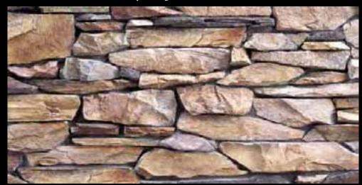
Square foot coverage for Canyon Ledge is based on installation with  $\frac{1}{2}$ " mortar joints. Page 25
